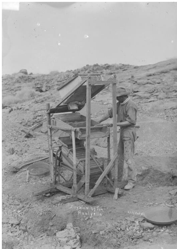
Figure 6-1: Dryblowing tin at Moolyella (ca. 1921)
